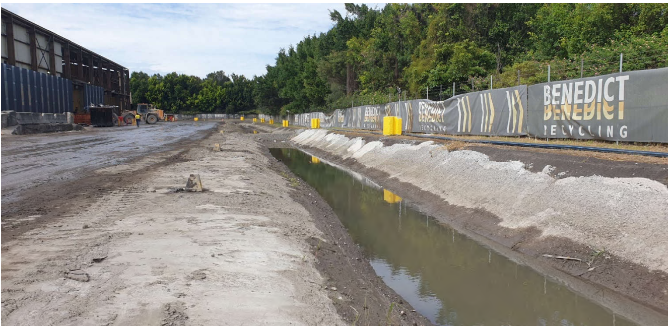
Photo 10 Main stormwater drain along western site boundary with gravel filters (basin walls) looking south
