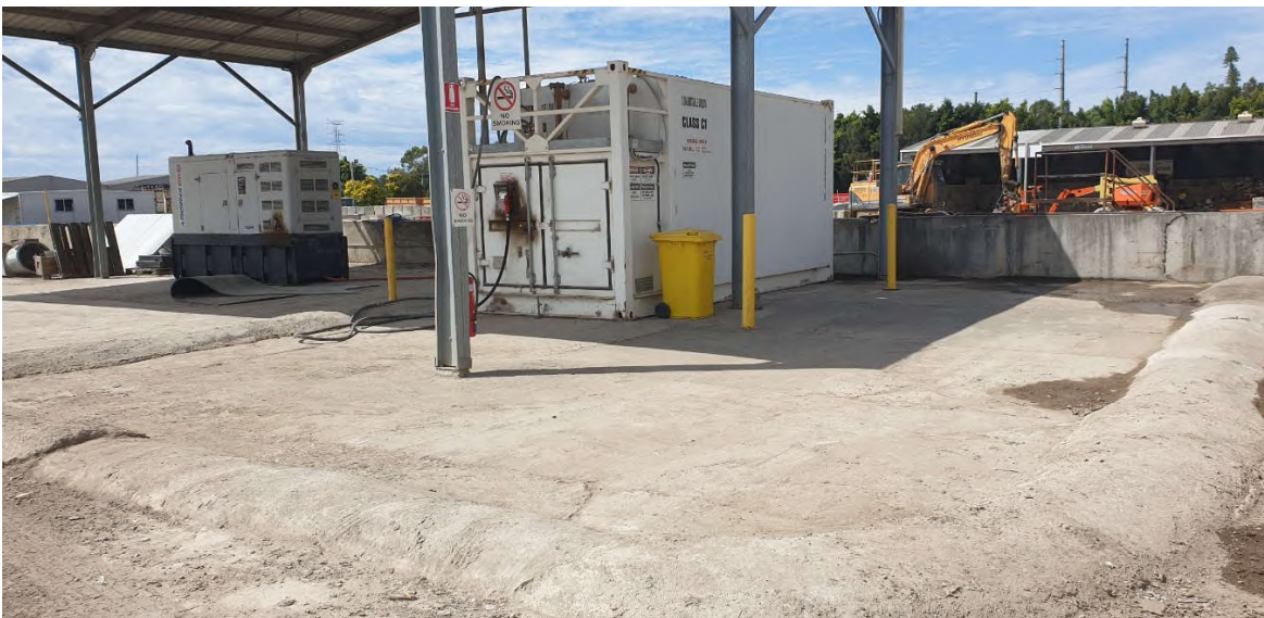
Photo 31 Generator and diesel fuel tank facility with external concrete bunding
