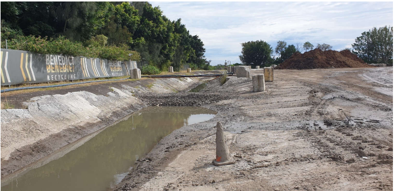
Photo 11 Main stormwater drain along western site boundary with gravel filters (Basin walls) looking north
