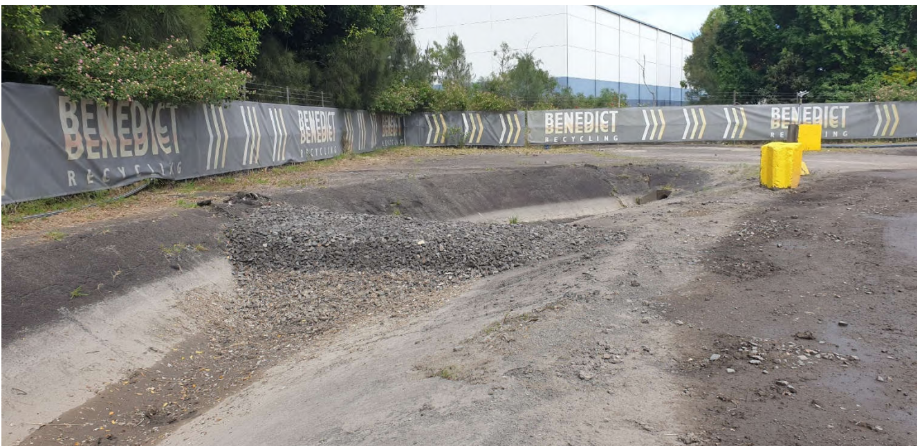
Photo 12 Main stormwater drain in SW corner of site with gravel filters (basin walls)
