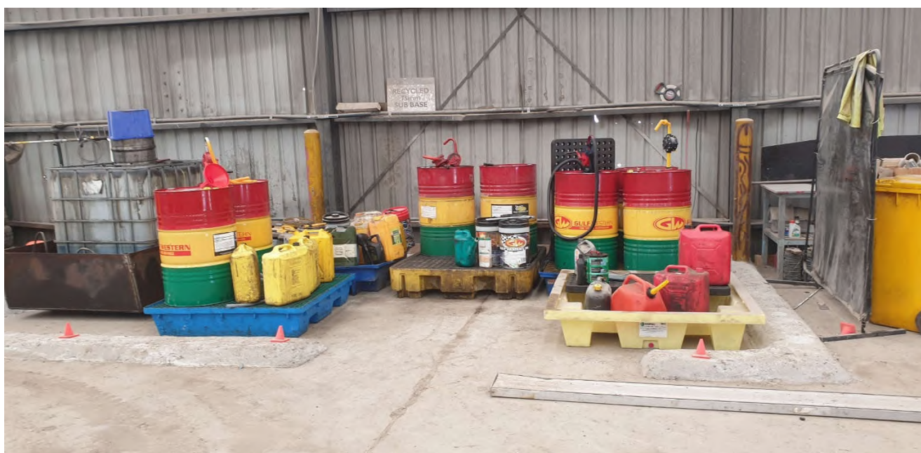
Photo 35 Minor chemical storage on bunded spill pallets in on-site workshop
