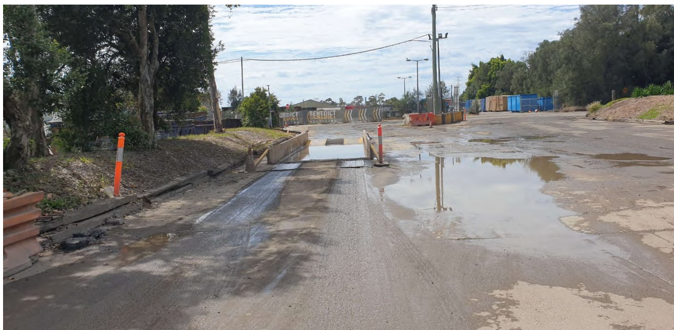
Photo 3 Wheelwash for trucks leaving site
