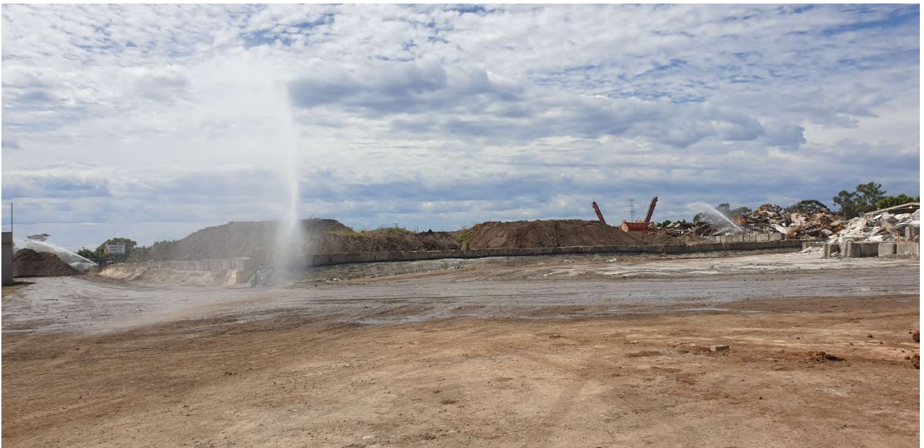
Photo 17 Dust suppression water sprays along northern boundary and central part of site viewed from NW corner of site
