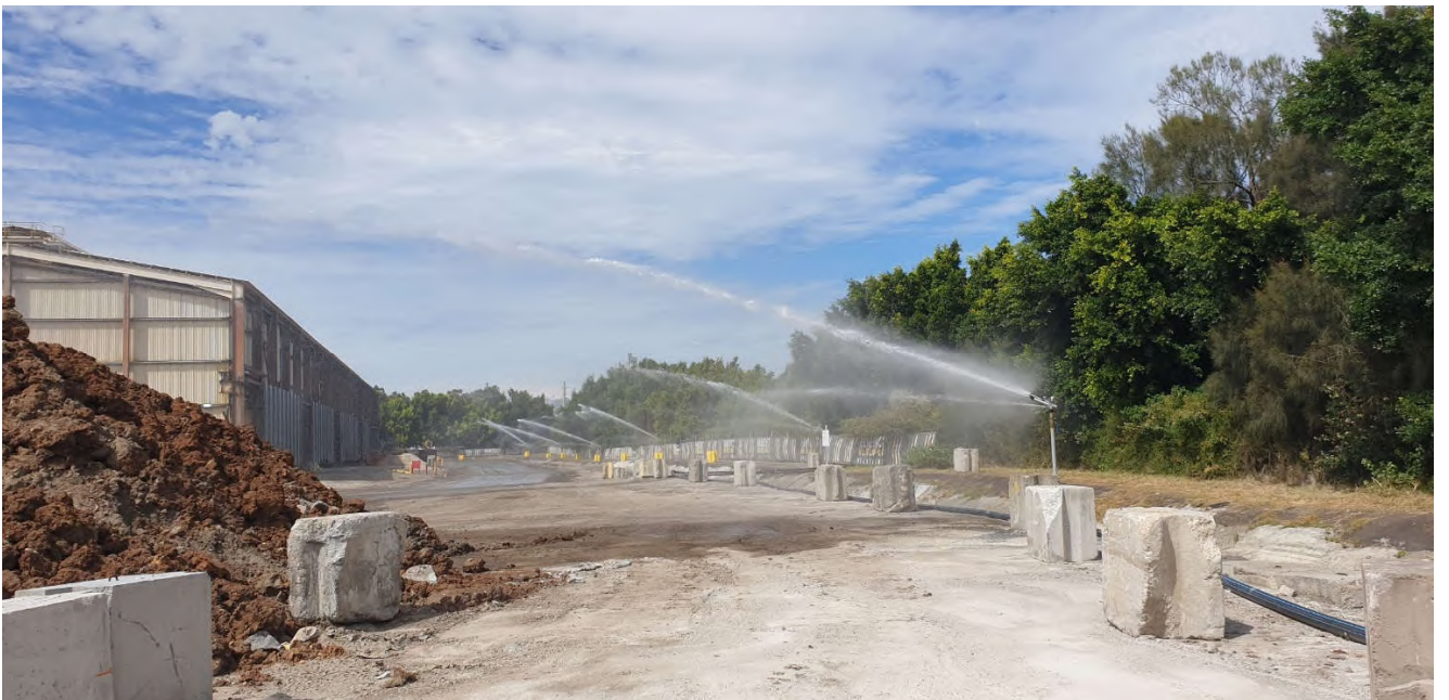
Photo 16 Dust suppression water sprays along western boundary viewed from NW corner of site
