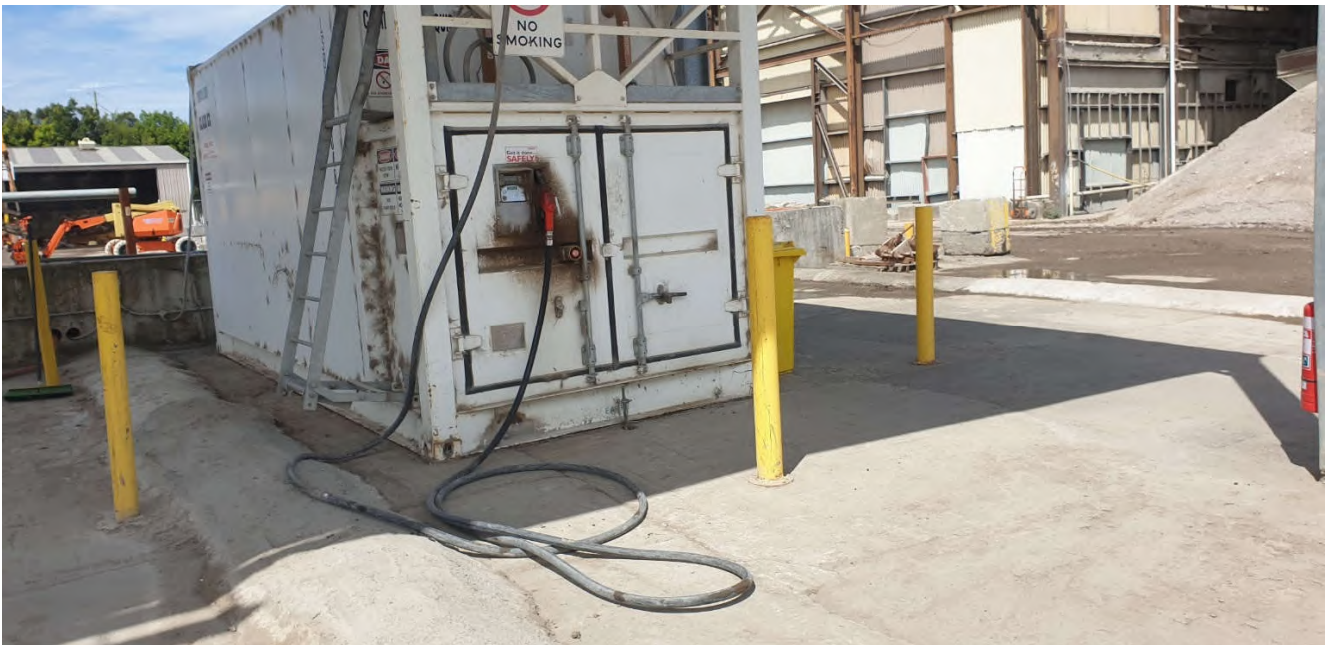
Photo 30 Double contained diesel fuel tank with external concrete bunding
