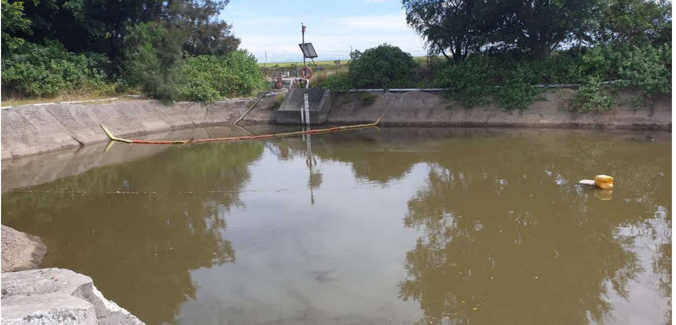
Photo 9 Final sedimentation basin at NW corner of site
