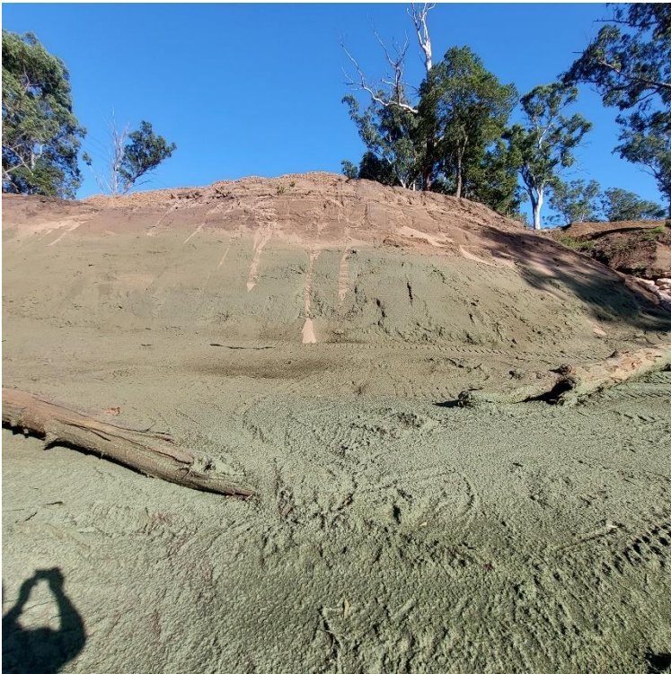
Photograph 5.20 Stage 8A/8B – hydromulching (dark green colouration) after extraction
