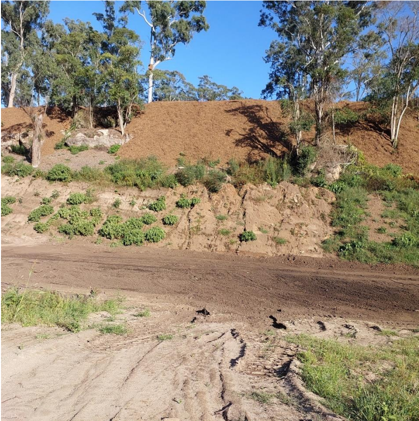
Photograph 5.17 Stage 8 Restoration Area 1/northern portion of Substage 8A (different locations) – Note mulch at top of slope, and some minor erosion at the base of the slope
