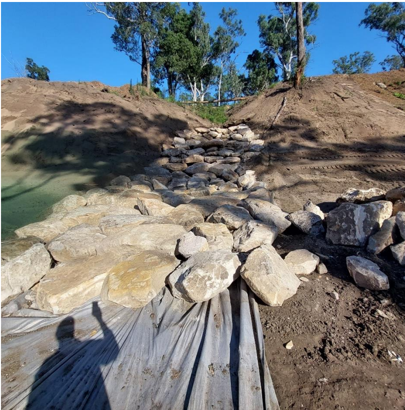
Photograph 5.19 Stage 8A/8B – Drainage line with scour protection works
