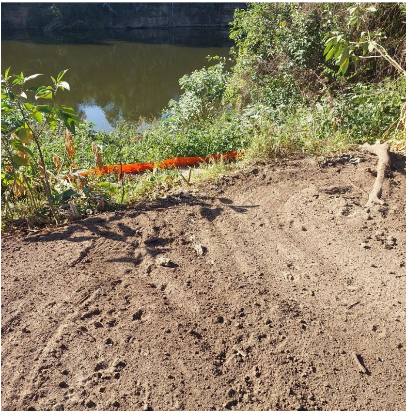
Photograph 5.18 Stage 8A – sediment fencing
