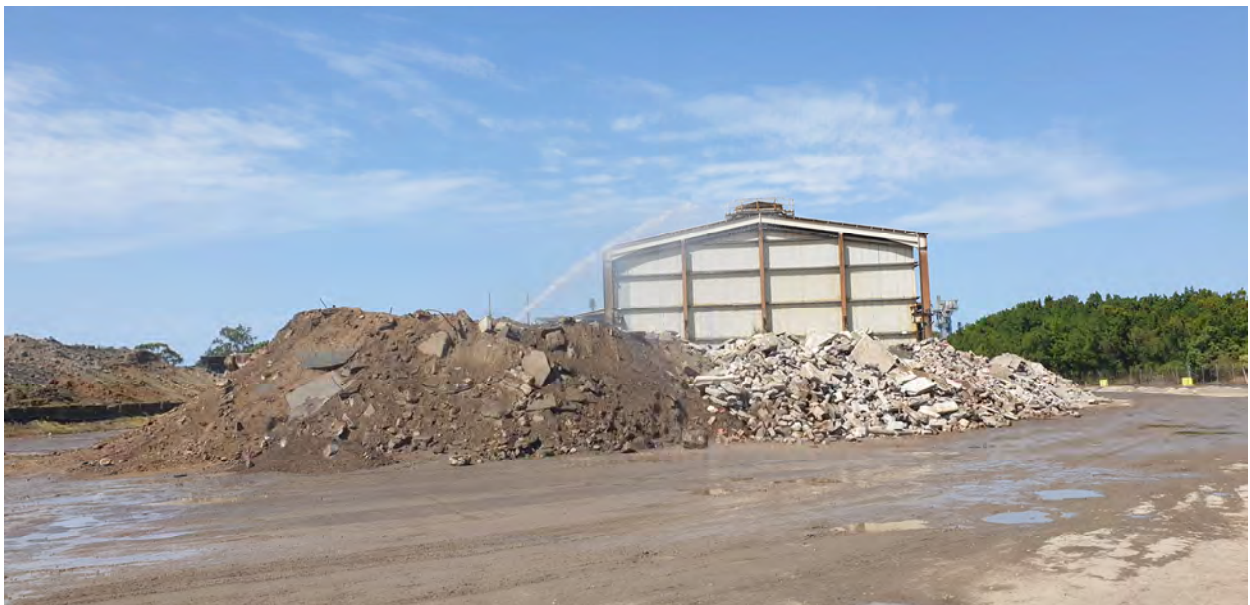
Photo 28 Water sprays in operation to suppress dust
