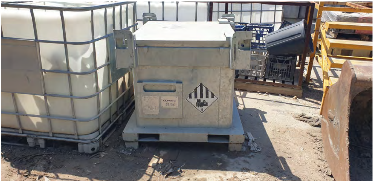
Photo 52 Storage of chemical waste on bunded pallets
