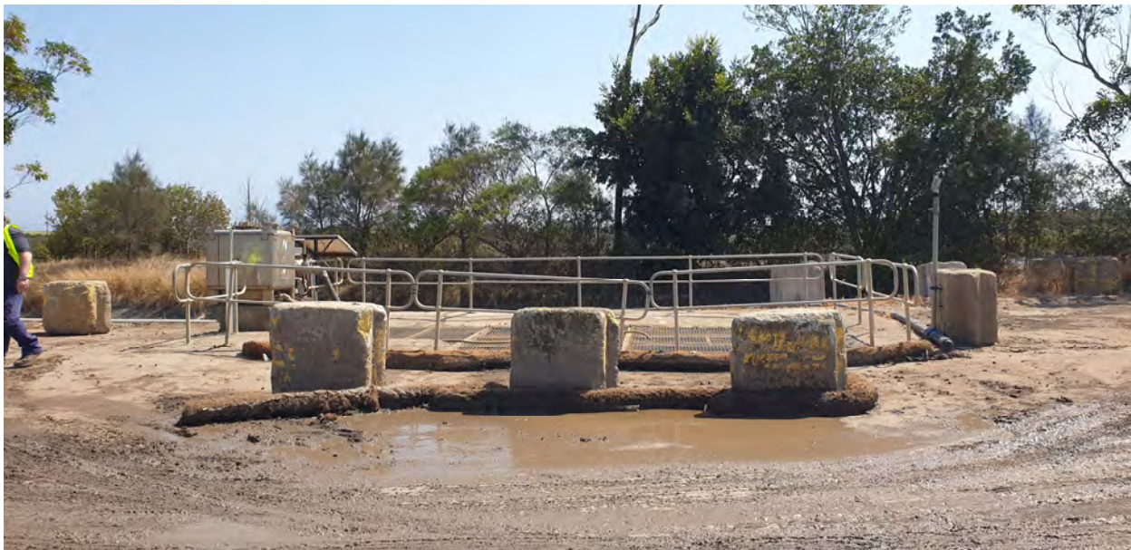
Photo 24 Two stage pit at northern end of Facility
