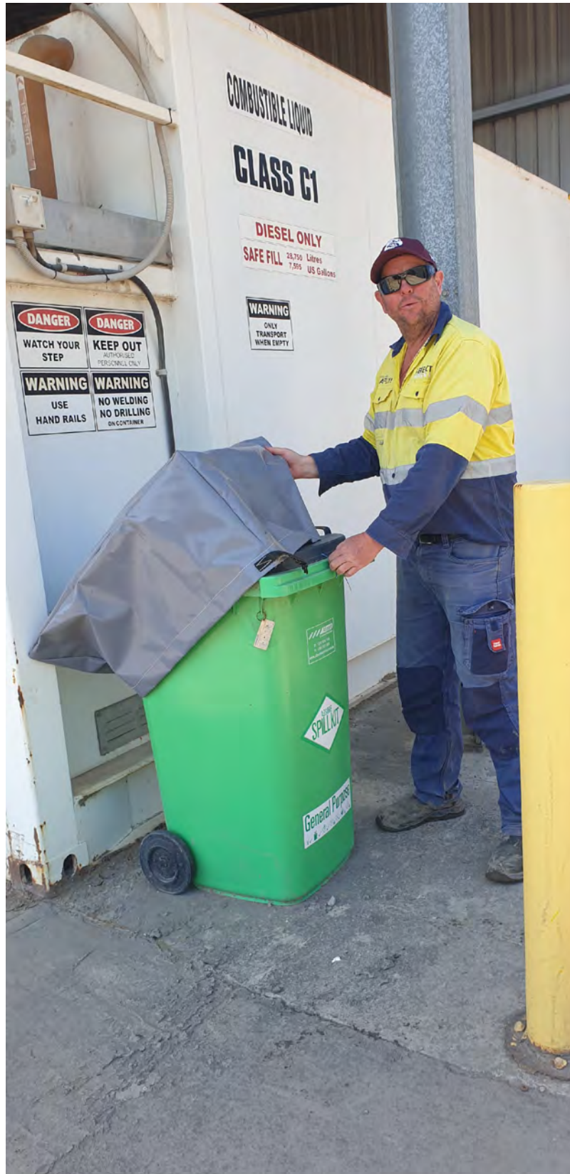
Photo 17 Spill kit in AST bunded area
