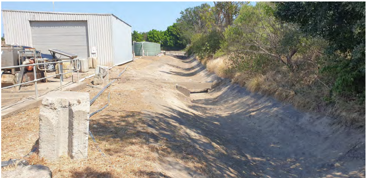
Photo 23 Concrete lined perimeter drain along northern side of Facility
