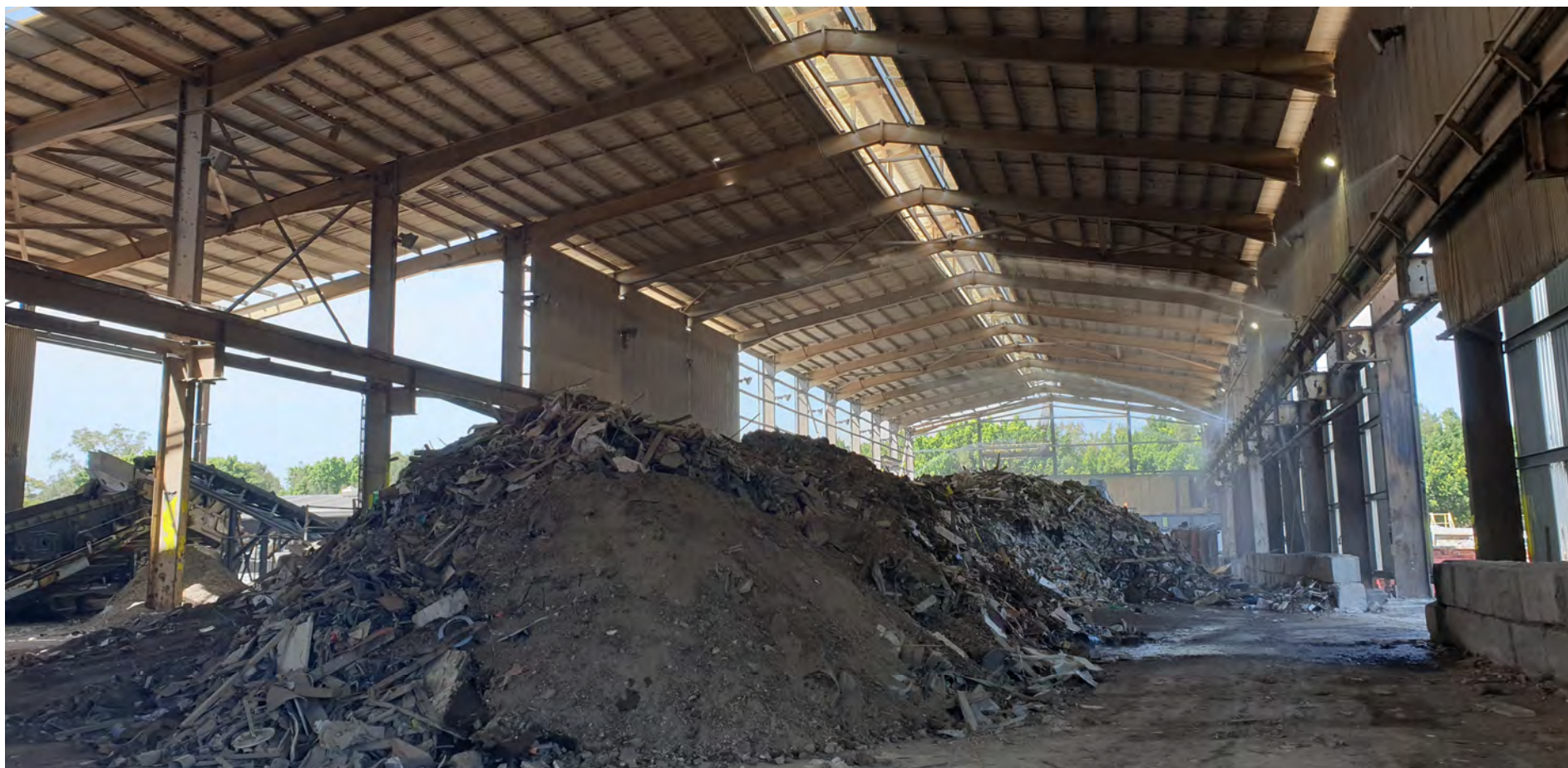
Photo 49 Stockpiled waste at northern end of main building prior to separation and with dust suppression sprays operating
