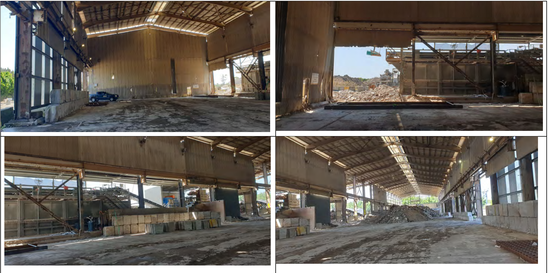
Photo 50 Main Processing Building looking south from northern end
