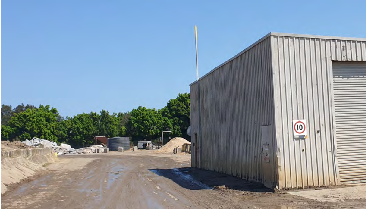
Photo 51 Stockpile height marker at northern end of Facility
