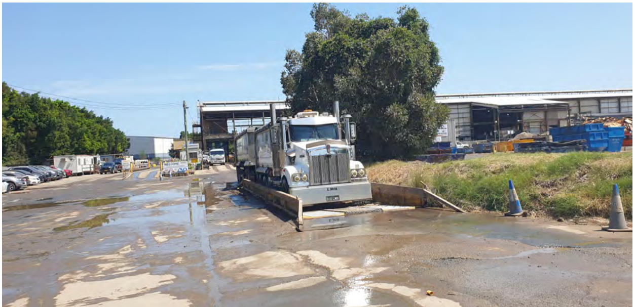
Photo 5 Wheel wash for trucks leaving site
