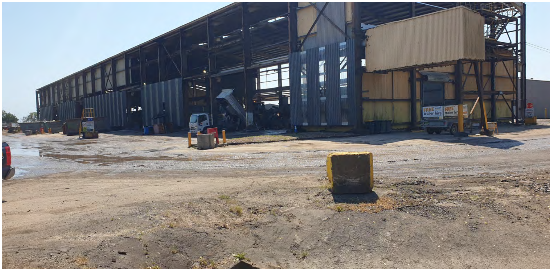
Photo 46 View of Main Processing Building
