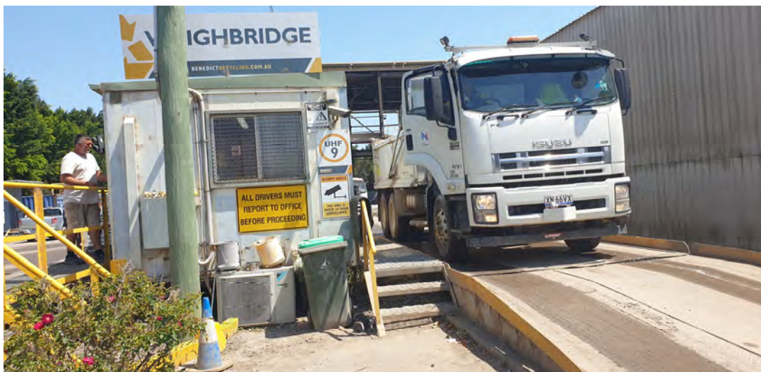
Photo 4 Automated weighbridge for incoming trucks and vehicles
