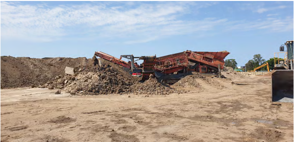
Photo 41 Screening plant in operation
