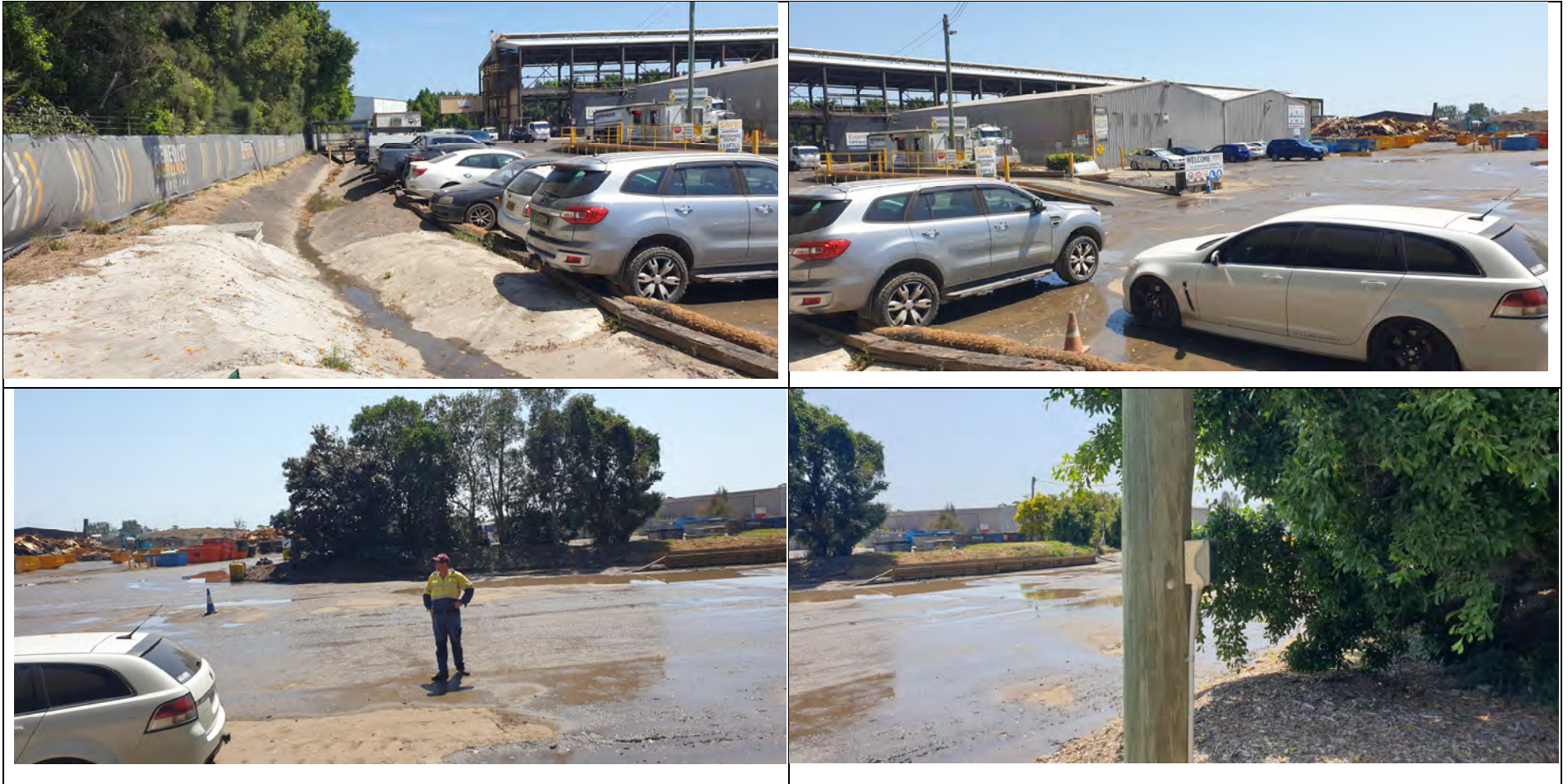
Photo 14 Sealed roads, kerb and gutters, fire mains and parking area at front area
