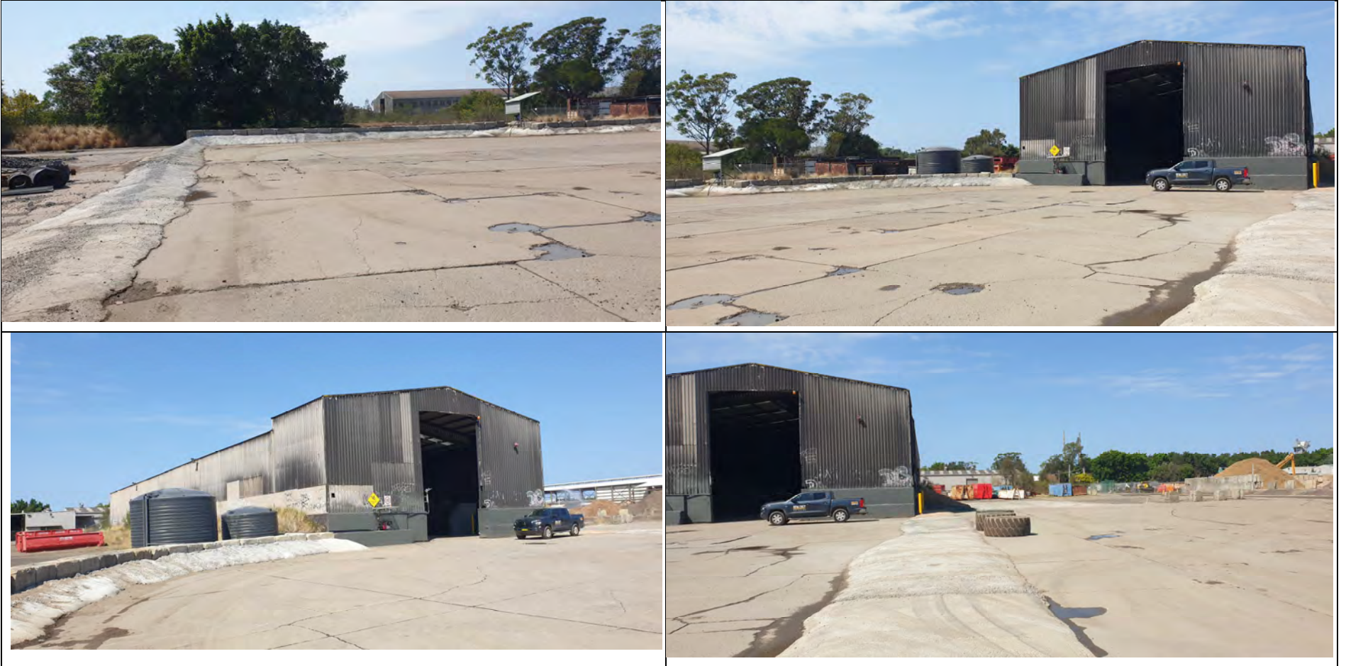
Photo 34 ASS treatment area – concrete slab and perimeter bunds
