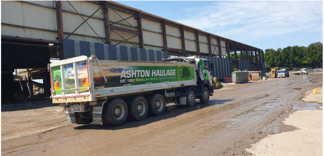
Photo 22 Dust suppression applied to western site road
