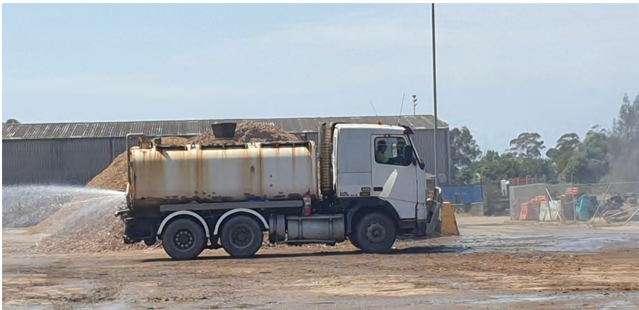
Photo 31 Operation of water cart to suppress dust in central part of Facility
