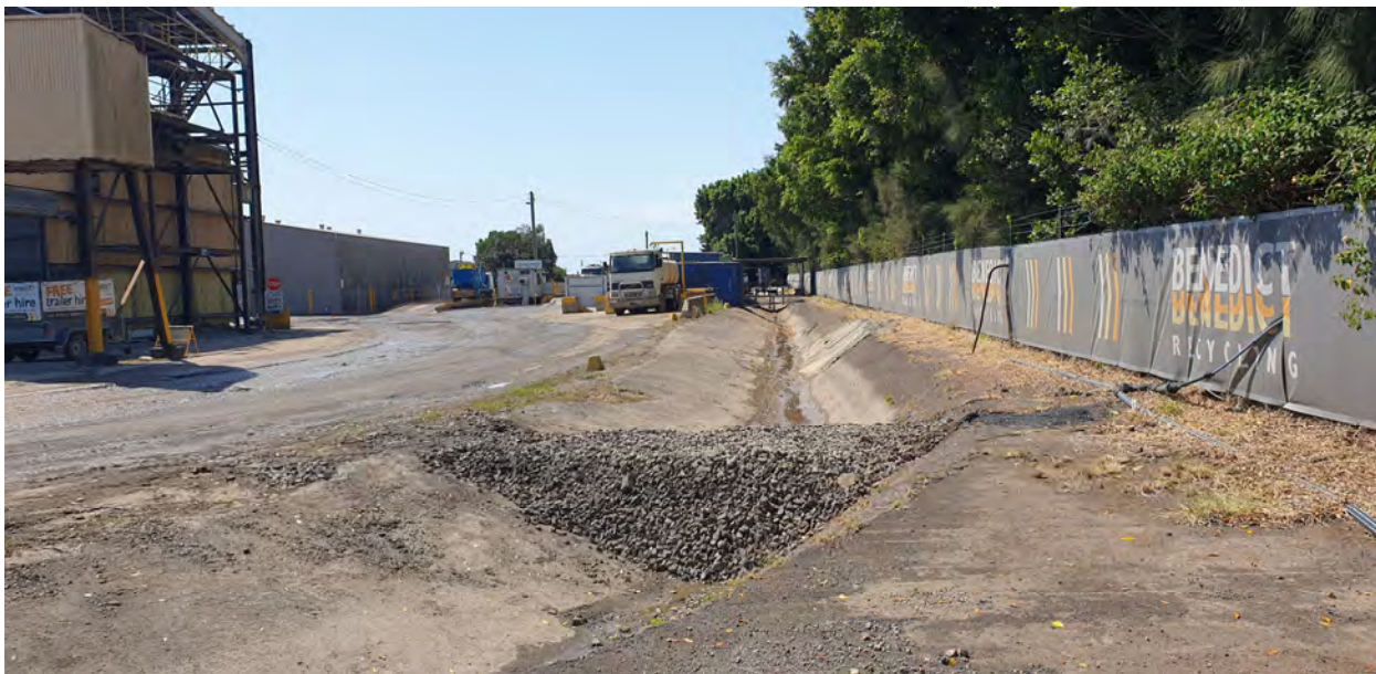
Photo 18 Concrete lined perimeter drain along southern side of Facility
