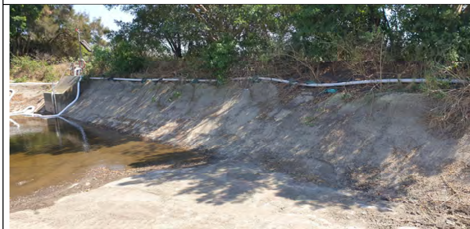
Photo 25 Final Sedimentation Basin at NW corner of site
