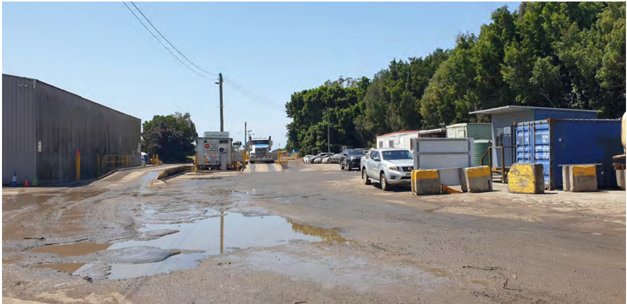
Photo 7 Admin area showing weighbridge, parking and site offices to right
