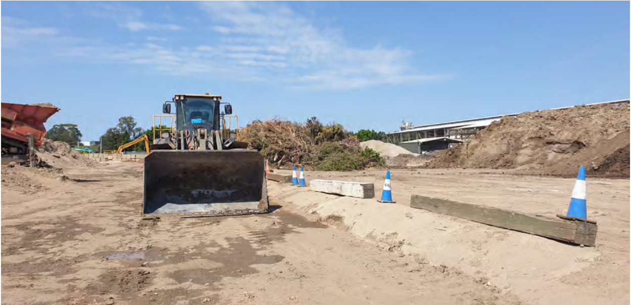
Photo 40 Front end loader used to feed screening plant with Mixed Waste and to manage screened materials
