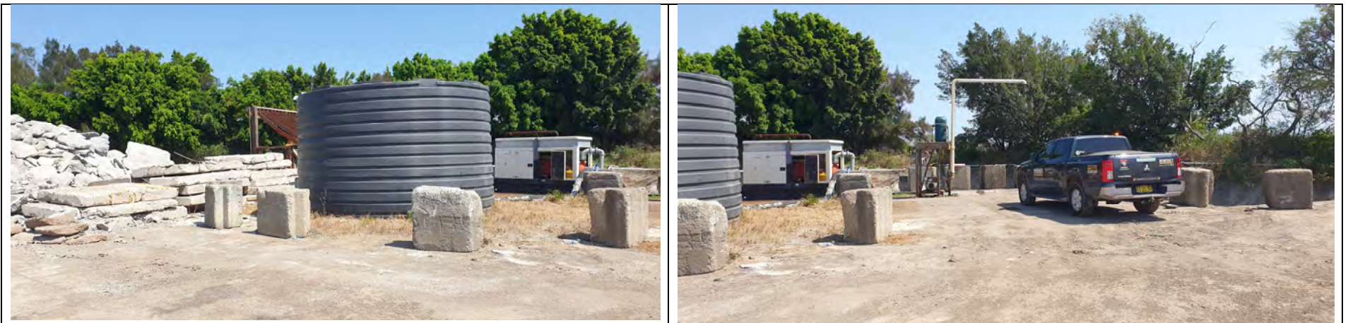
Photo 29 Water filling station for water cart located in northern end of Facility
