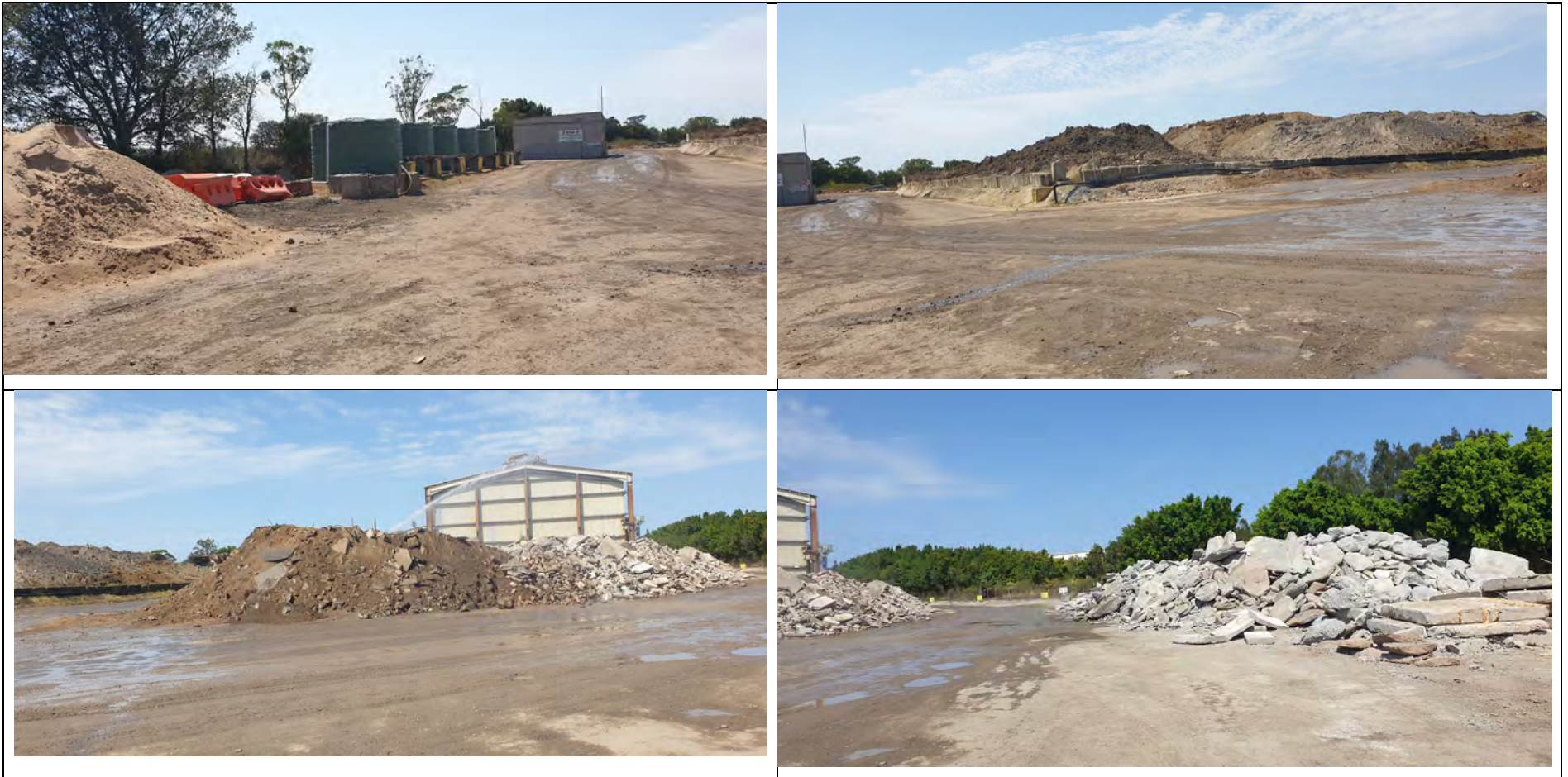
Photo 42 Waste processing area in northern part of Facility
