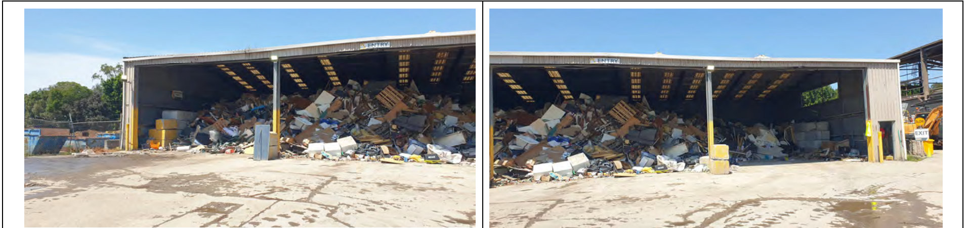
Photo 43 Undercover unloading area for Domestic Waste
