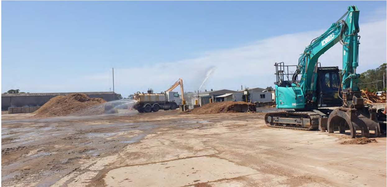
Photo 32 Operation of water cart and water sprays to suppress dust
