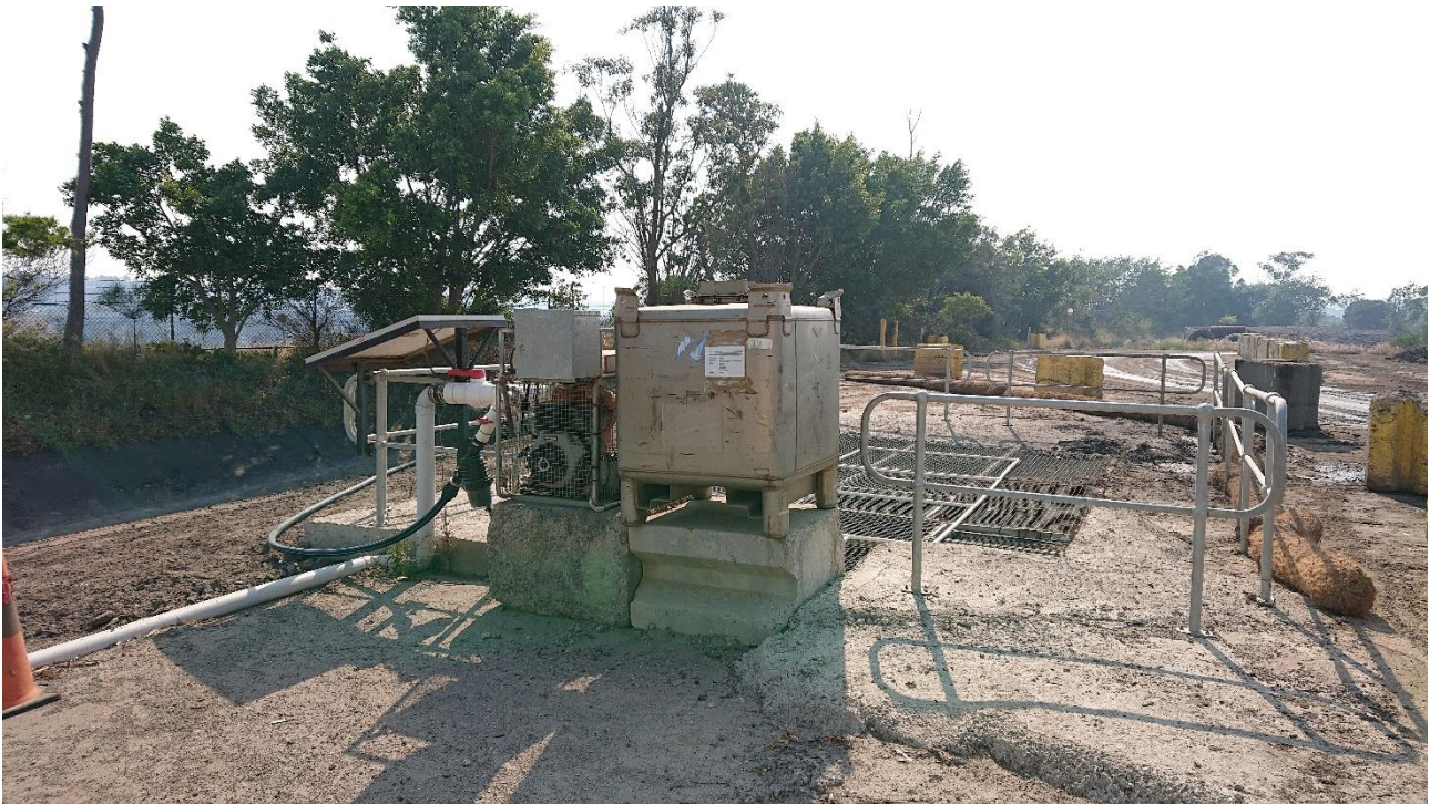
Photo # 12 - Wastewater Sump, pumps and treatment system
