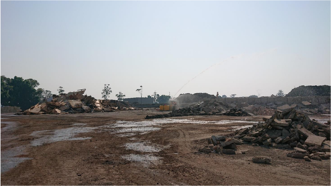
Photo # 3 - Timber (pallets) and concrete stockpiles
