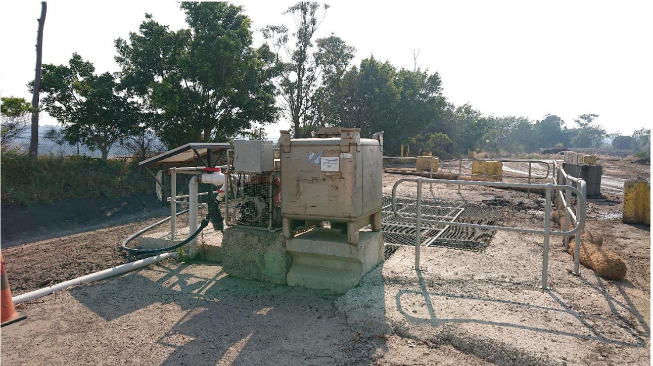
Photo # 12 - Wastewater Sump, pumps and treatment system
