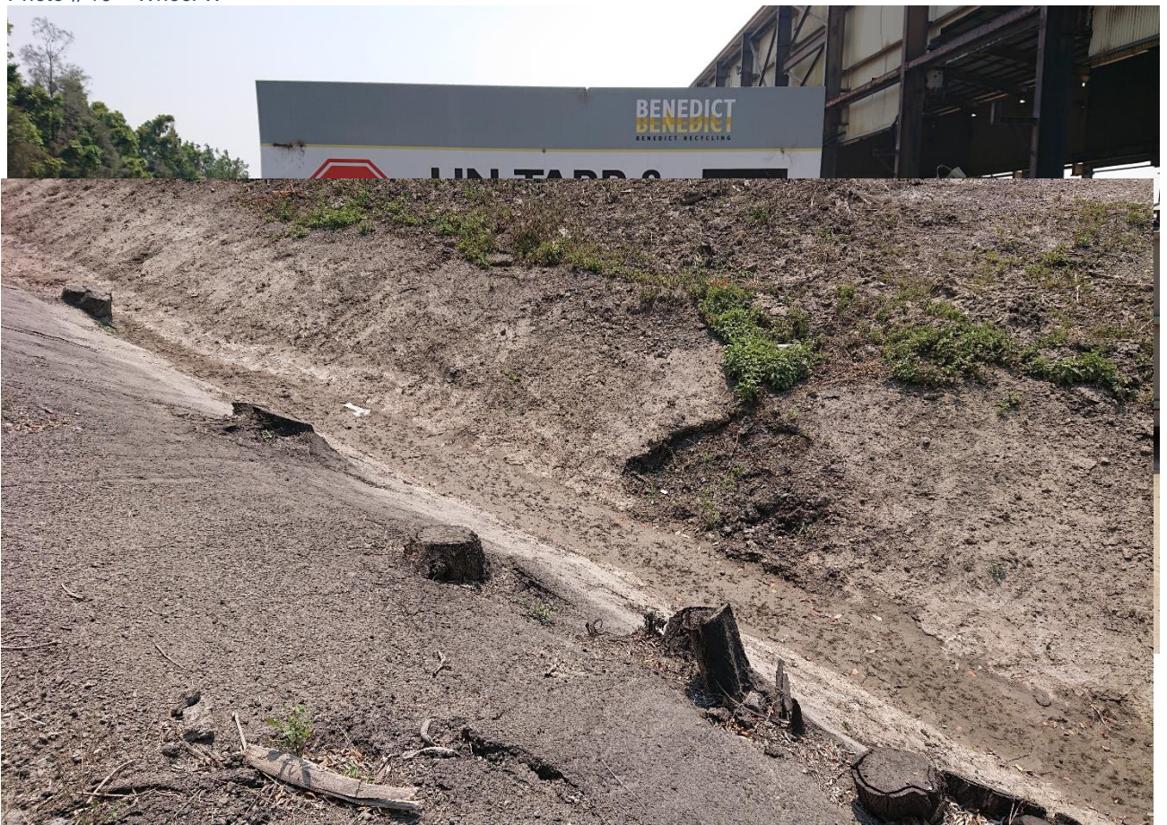
Photo # 9 - Perimeter Drain
