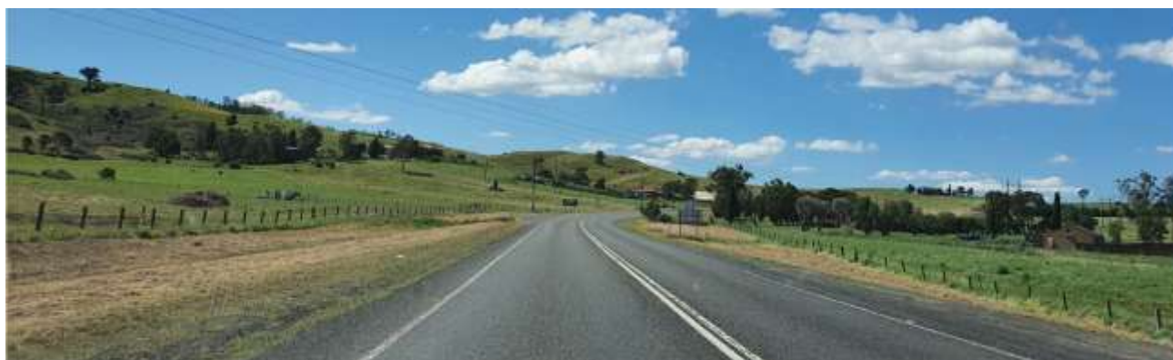
Plate 3.1 Menangle Road (looking north, south of the site)
