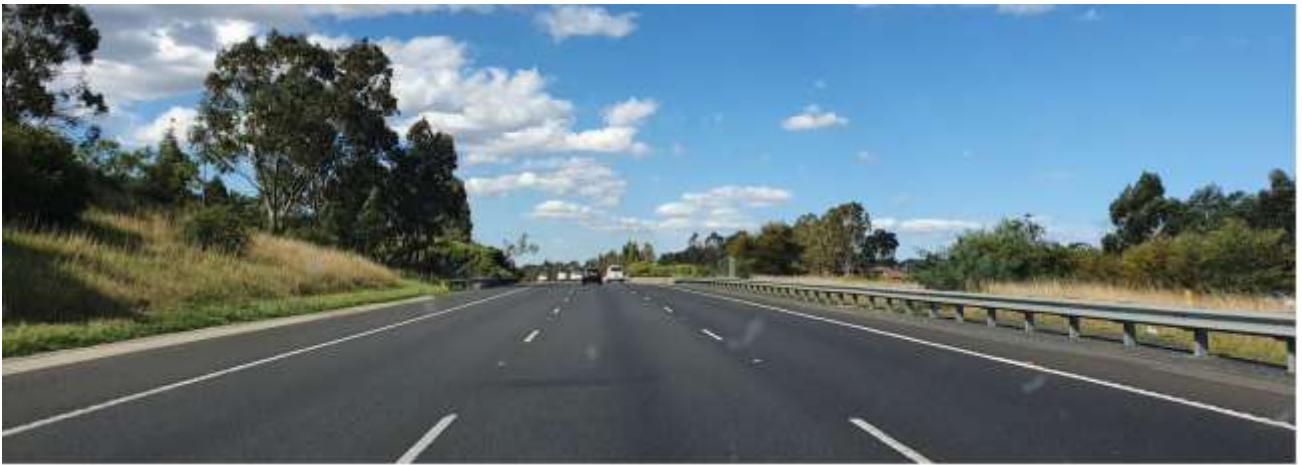
Plate 3.5 Hume Highway (looking north, near Menangle Road)
