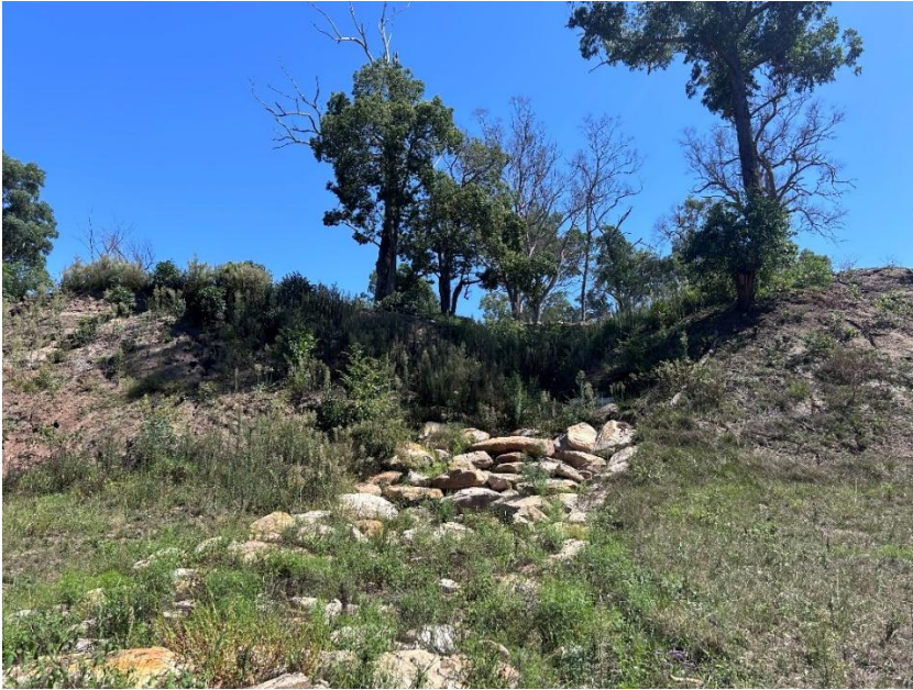
Photograph A.17 Stage 8A/8B drainage line with weed infestation
