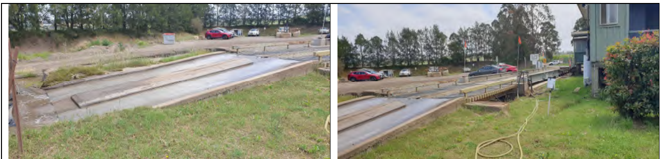
Photo 4 Wheelwash for trucks leaving site located before weighbridge
