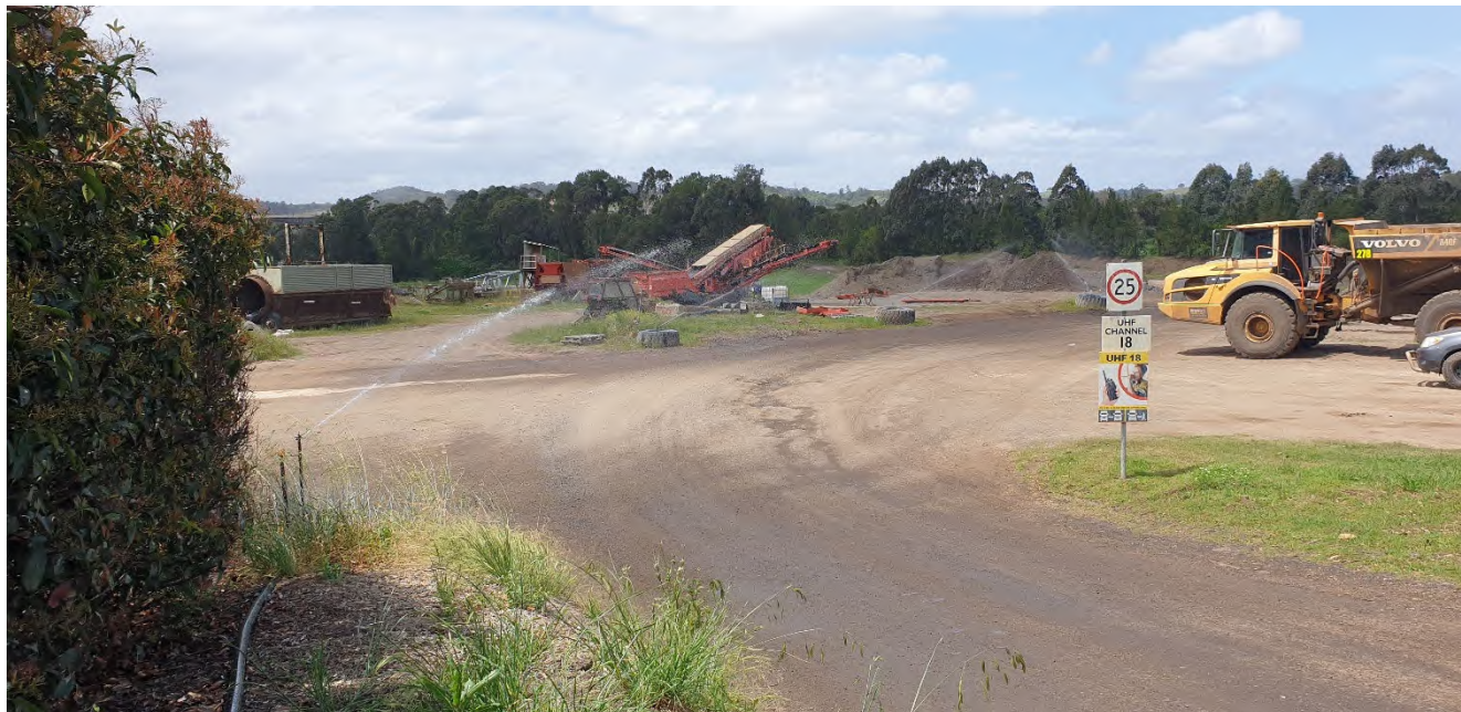
Photo 8 Automated dust suppression system at equipment laydown area near site office
