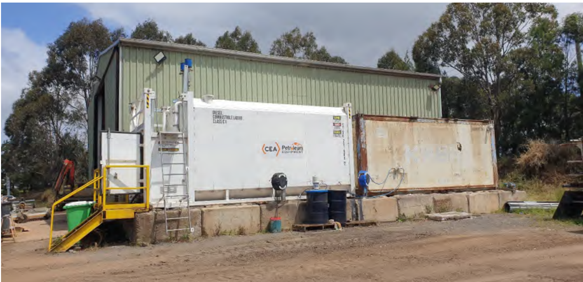
Photo 7 Self banded diesel fuel storage tanks
