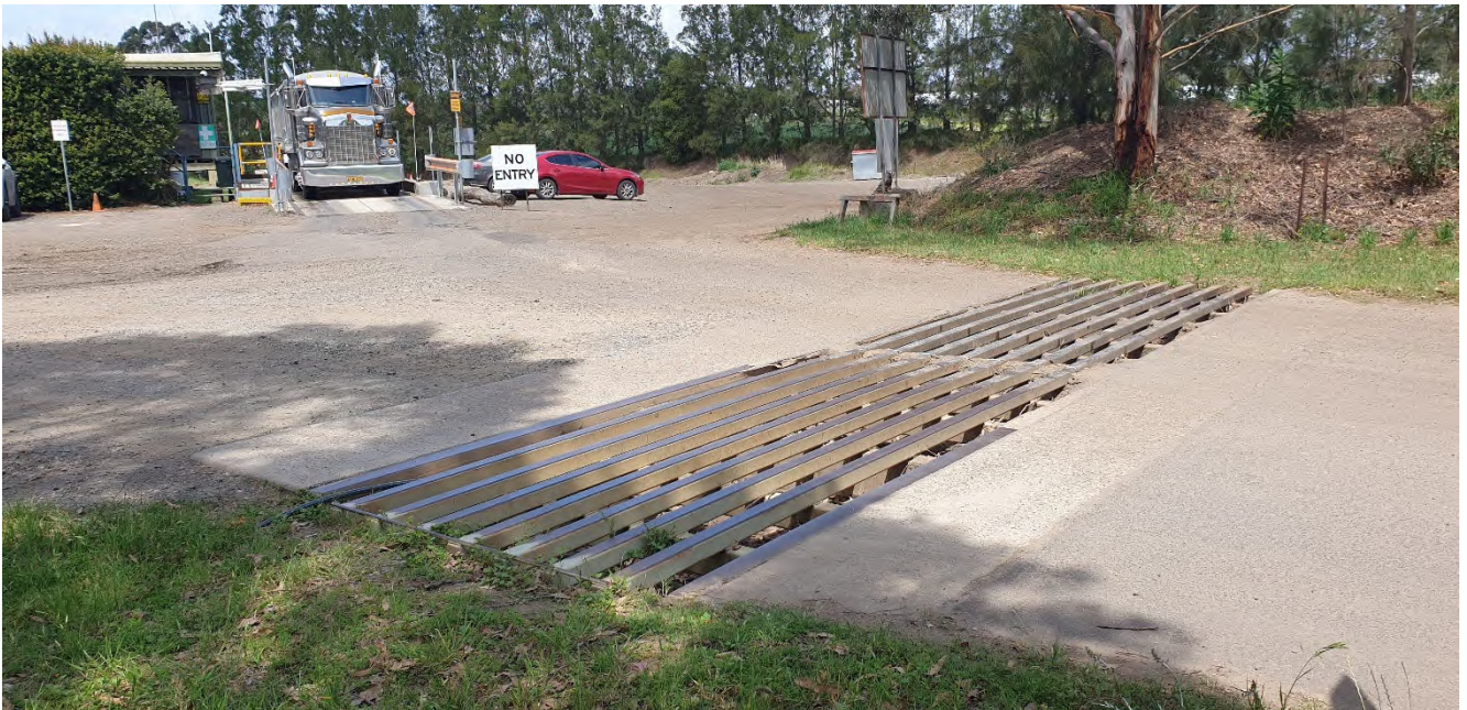
Photo 2 Rumble grid near site entrance / exit with weighbridge and office in background
