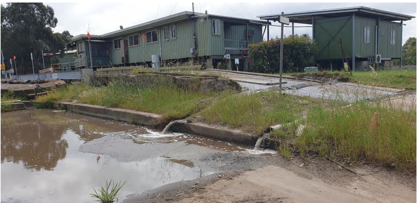
Photo 5 Wheelwash water holding pond
