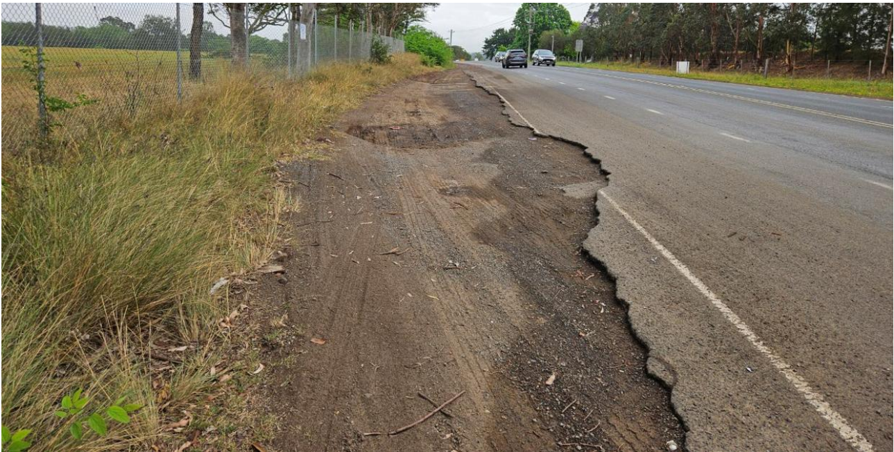
Plate 4.4 Edge of pavement is breaking up at opposite side of the Benedict site access
