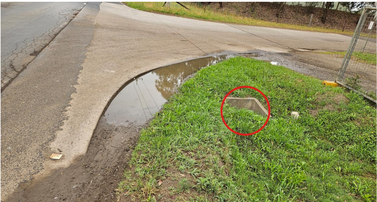
Plate 4.5 Water ponding on the left-hand side of the driveway
