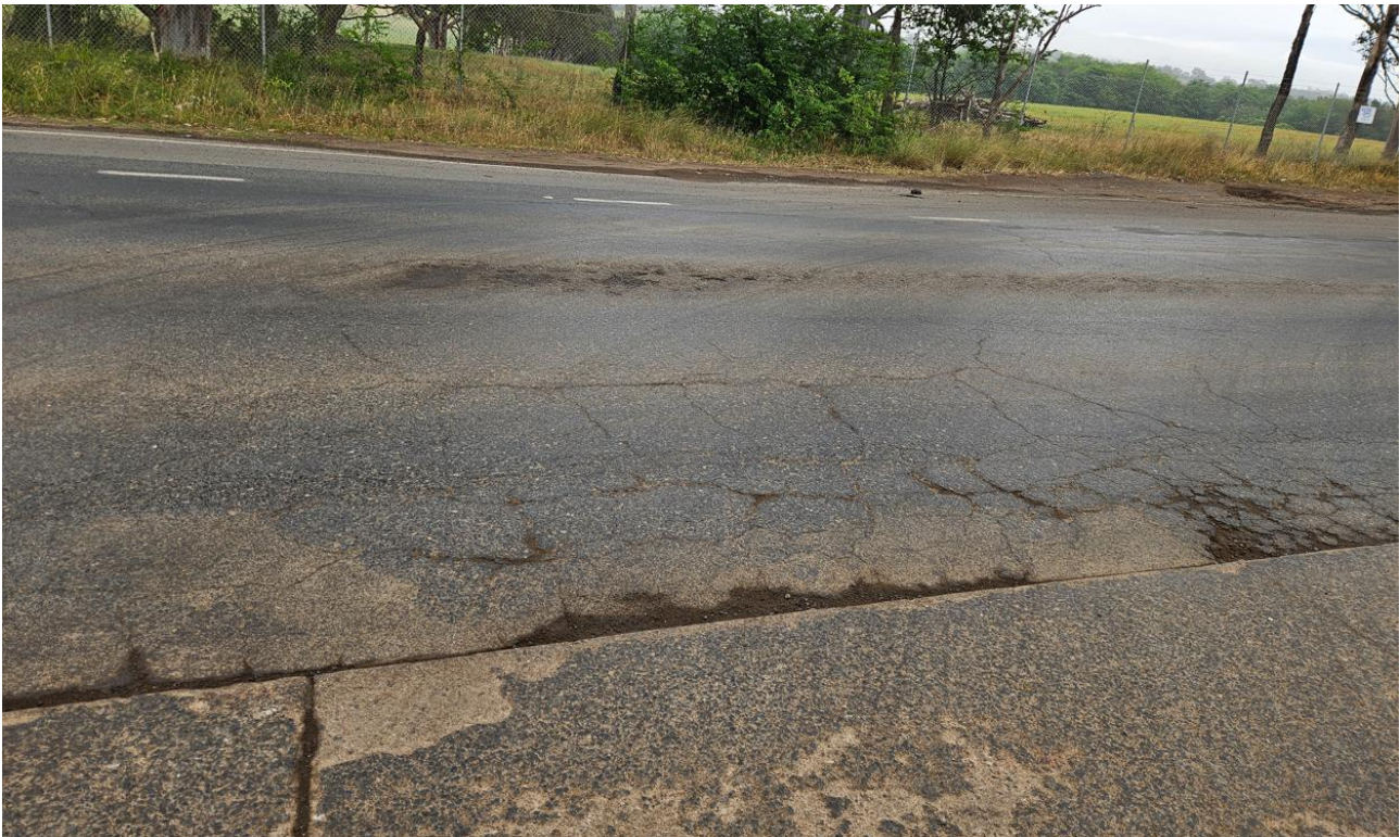
Plate 4.3 Pavement cracks on Menangle Road at the site access
