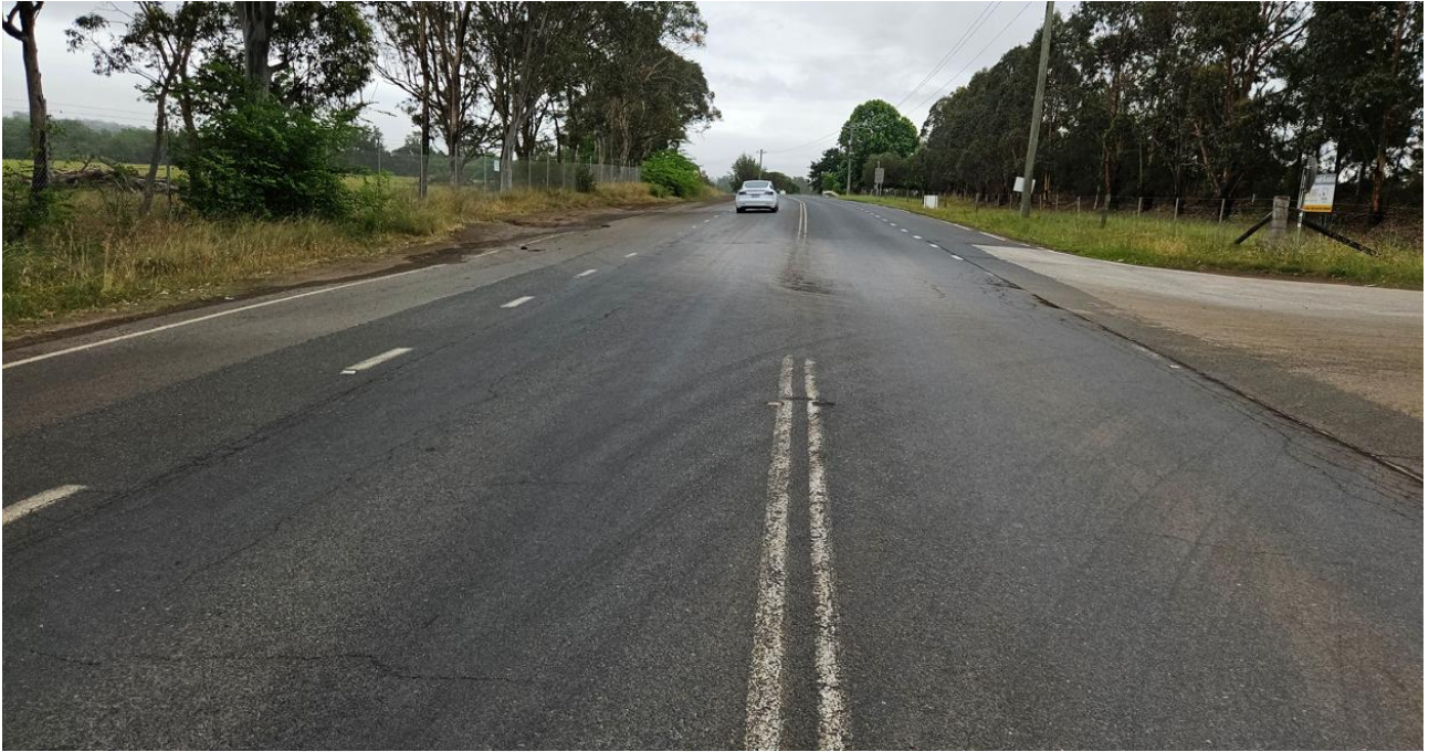
Plate 4.6 Faded line marking and missing pavement markers on Menangle Road
