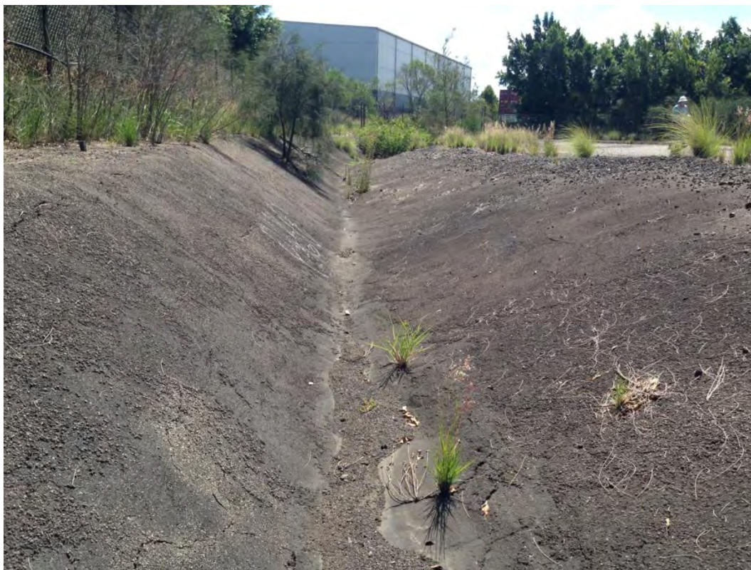
Photograph 2.17 Perimeter drain at the south end of the site (almost two metres deep at this point)
