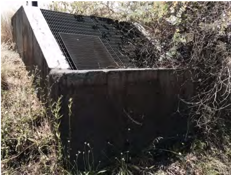
Photograph 1.6 Sedimentation pond discharge point in north-west of the site
