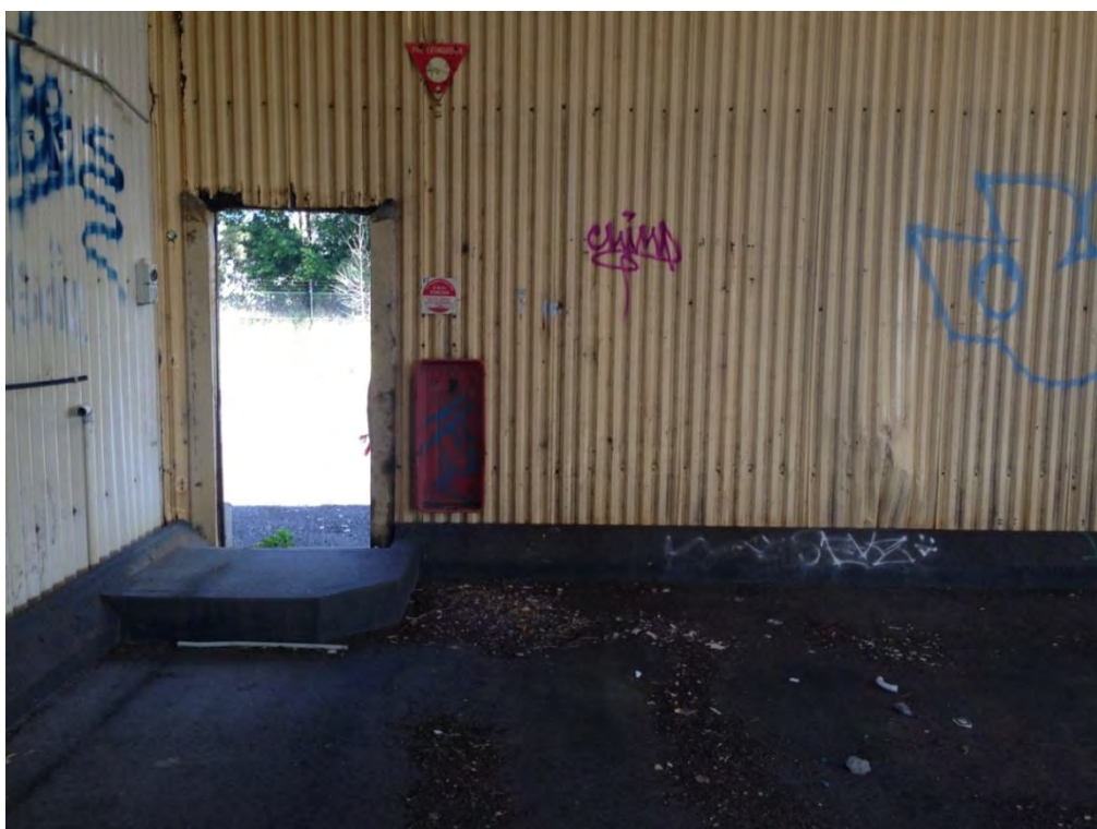
Photograph 2.4 Interior of main processing shed showing bunding around access door
