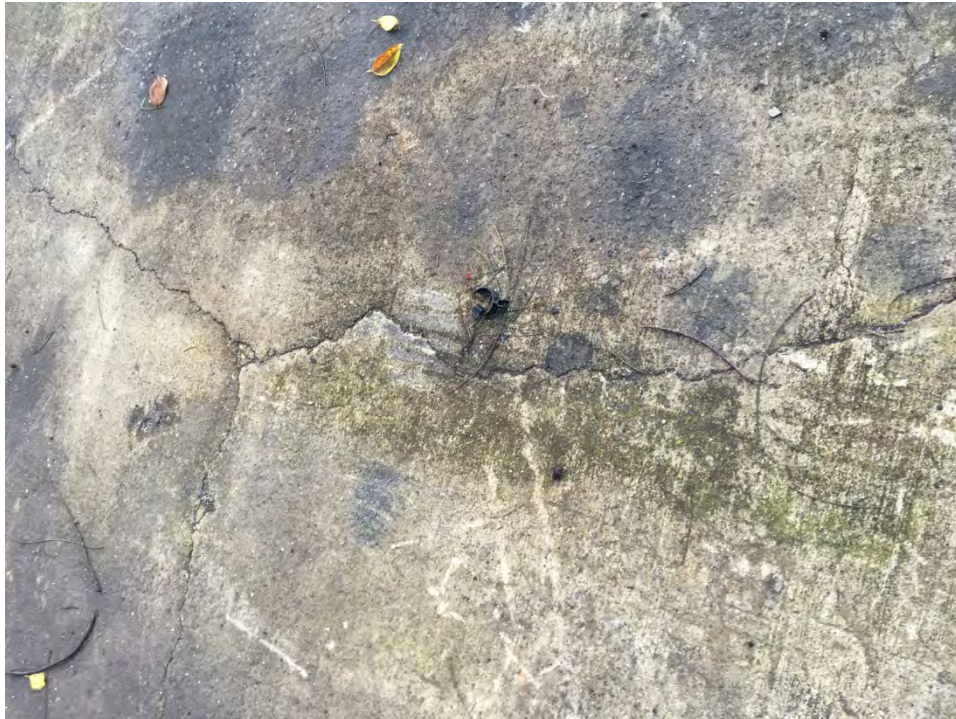
Photograph 3.2 Cracks in the concrete seal
