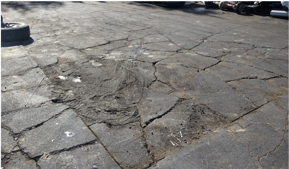
Photograph 3.4 Cracks in concrete slab
