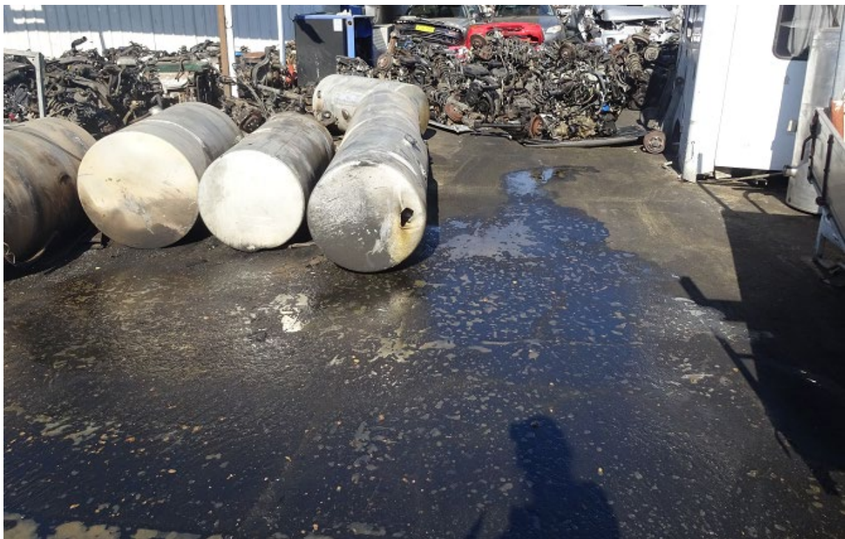
Photograph 3.1 Oily sheen on concrete slab
